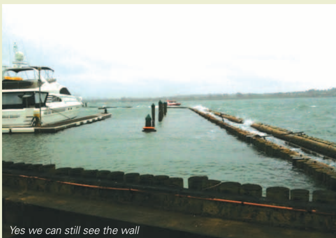
A Pier attenuator doing its job
